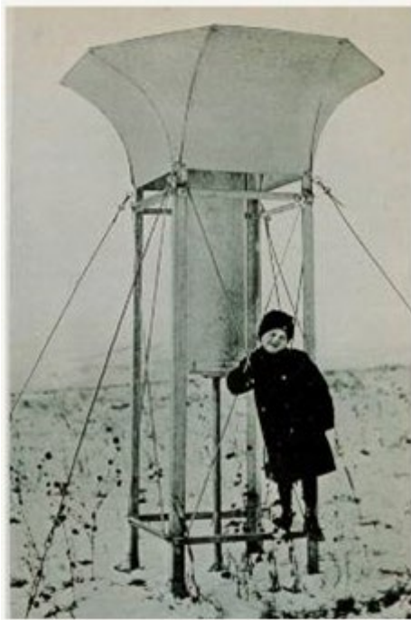
Figure 3.3.12-2: Shielded snow gauge used in the pacific northwest to register snowfall, 1917
