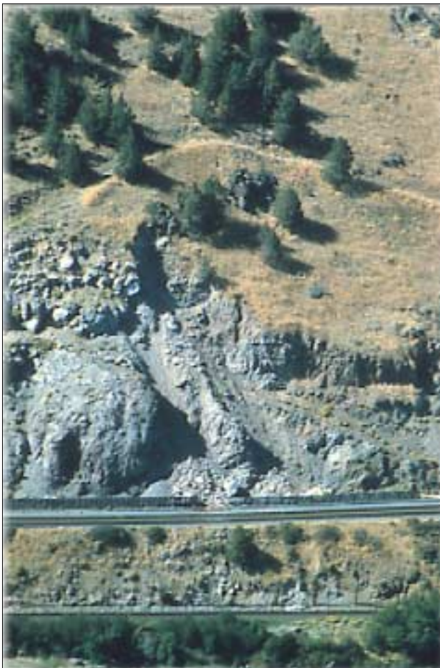
This landslide was triggered by a 1993 Klamath Falls earthquake and caused one of the two deaths from that event. (photo courtesy Oregon Department of Geology and Mineral Industries)
