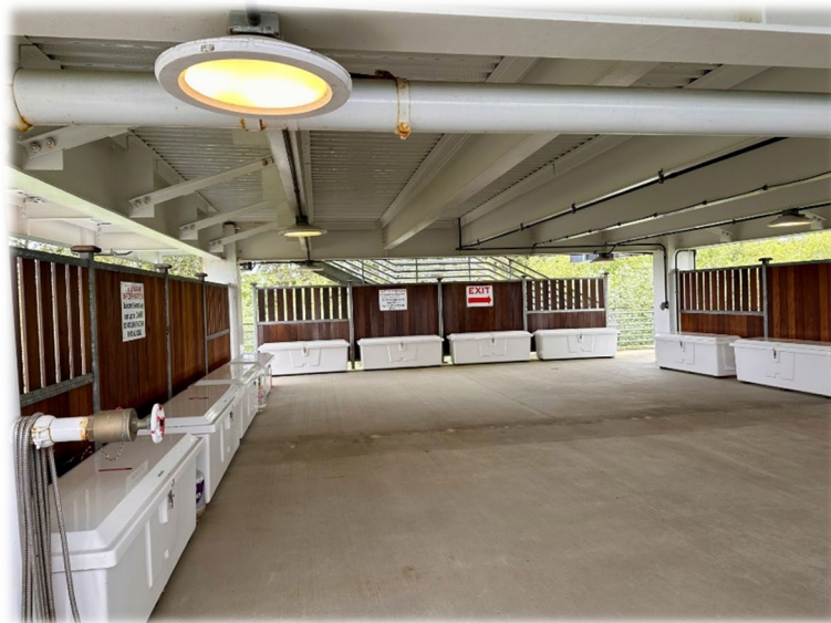
Figure 26: Tokeland Tower (Auntie Lee Tower) first floor
