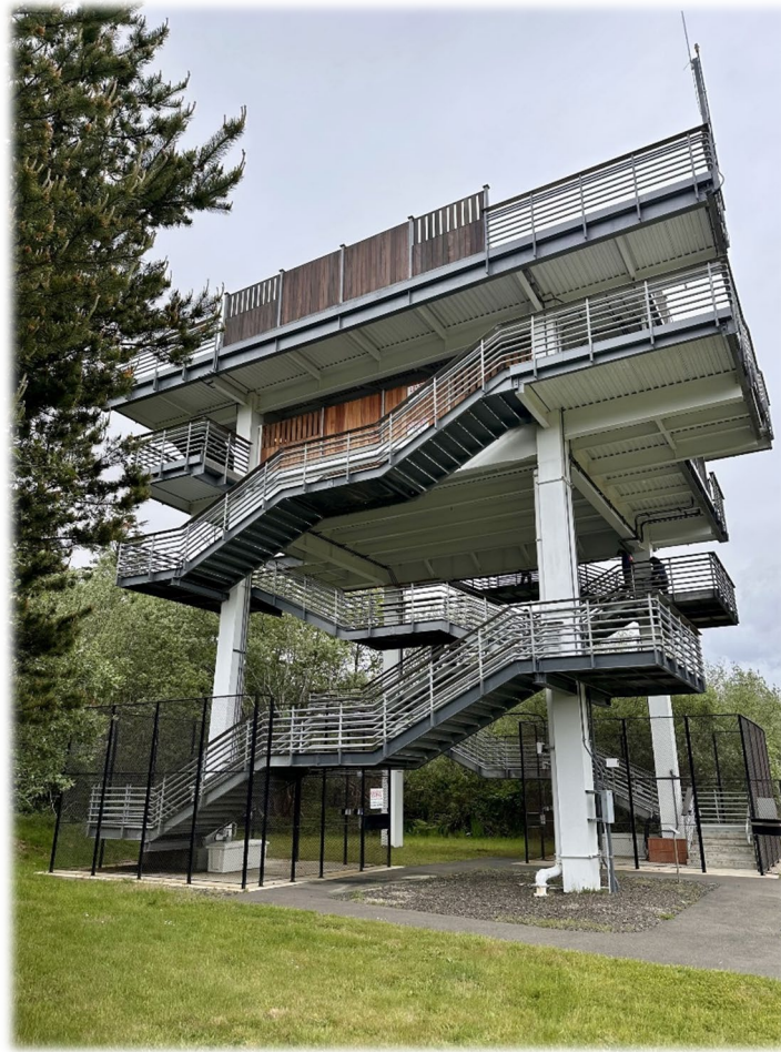
Figure 25: The Shoalwater Bay Indian Tribe’s tsunami vertical evacuation tower in Tokeland, Washington—the first free-standing structure of its kind in the United States.
