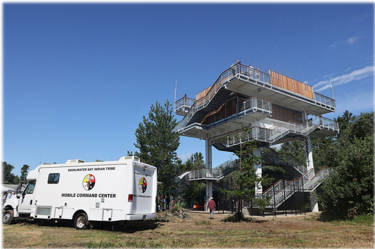
Figure 18: Shoalwater Bay Tribe Tsunami Tower – Tokeland, Washington. Photo Credit: Washington Military Department.
