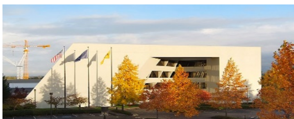
OGEC's office is located in the Morrow Crane Building
