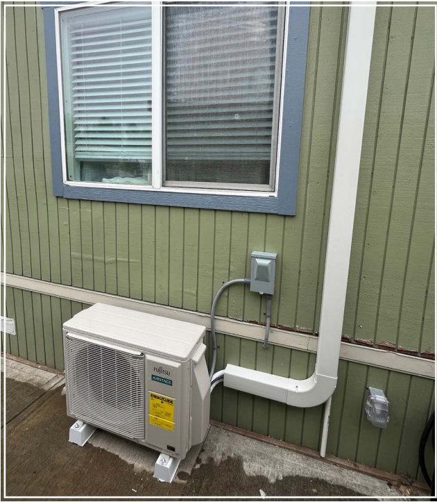
Installed Wood Village Green Mobile Home Park mini-split
