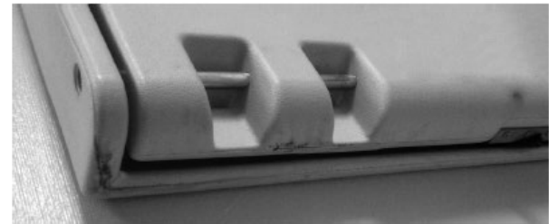
Figure 2. Photograph of underneath the diaper changing station involved in this outbreak, which had allegedly been cleaned twice by janitorial staff. This level of soiling was consistently viewed in public restroom diaper-changing stations.
