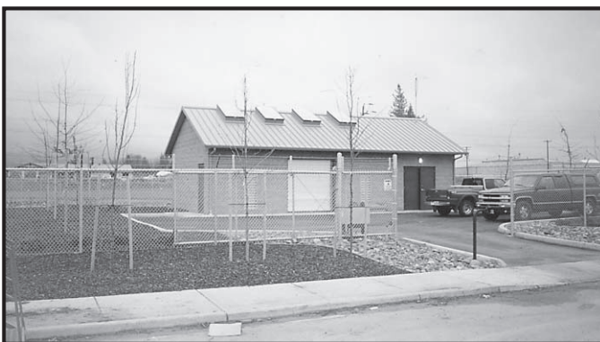
Regional Pump Station
