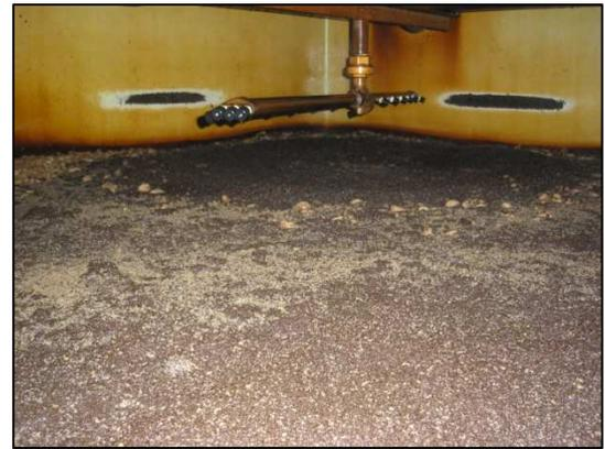
fouling of the filter media. Mud ball formation is heightened by the use of polymers such as coagulants or filter aids. Mud balls can usually be detected as they grow to the size of a pea, although they can grow to as large
