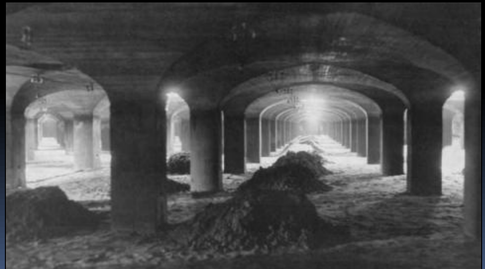
US Army Corps of Engineers photo of Washington DC McMillan Water Filtration Plant, a 25-acre, 75 MGD slow sand plant in use from 1905 – 1985
