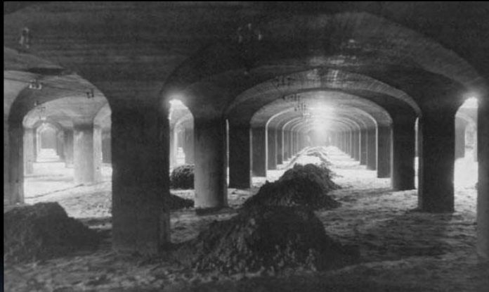
US Army Corps of Engineers photo of Washington D.C. McMillan Water Filtration Plant, a 25-acre, 75 MGD slow sand plant in use from 1905 – 1985 (replaced by rapid sand plant). Eliminated typhoid epidemics in the City.
