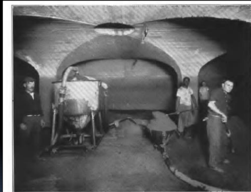
J. TORRESDALE PLANT, SHOWING METHOD OF CLEANING WITH NICHOLS SEPARATOR.
