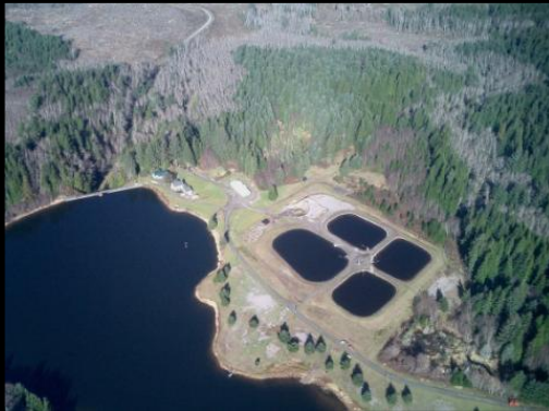
Astoria, OR 5 MGD plant (photo taken by Frank Wolf)
