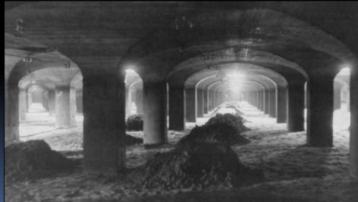
US Army Corps of Engineers photo of Washington DC McMillan Water Filtration Plant, a 25-acre, 75 MGD slow sand plant in use from 1905 - 1985
