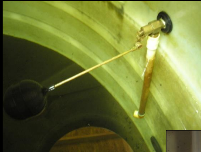
Float control valve. Camp Yamhill in Yamhill Co. Oregon. 2012.
