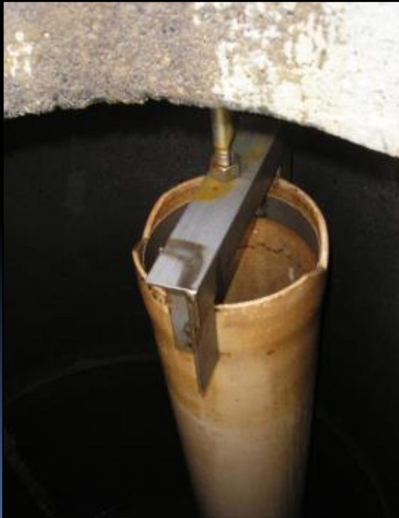
Telescoping Valve. City of Cannon Beach in Clatsop Co. Oregon. 2013.
