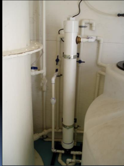
Privately owned slow sand filter & limestone calcite contactor Photos by Stephen Tanner
