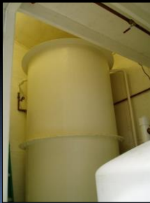
Privately owned slow sand filter & limestone calcite contactor Photos by Stephen Tanner
