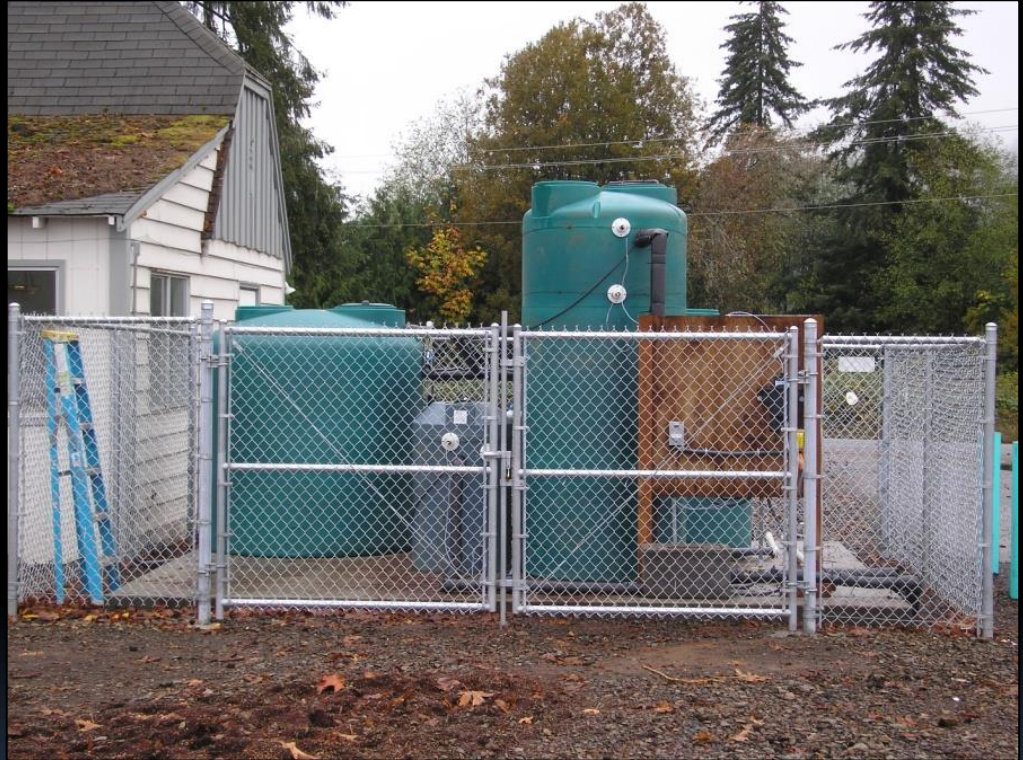
2009. Jewell School District #8, OR. "Blue Future" covered filter (left) and raw water control tank (right)
