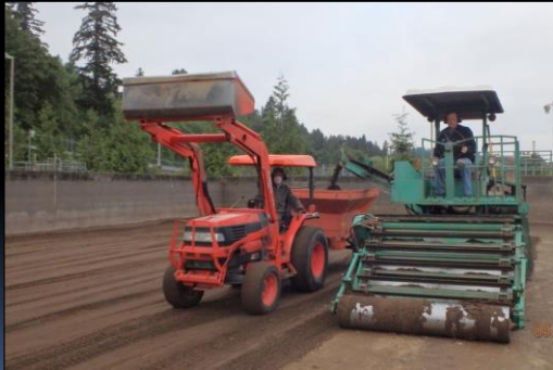
2013. North Clackamas County Water Commission, OR. SSF Cleaning (photo taken by Chris Johnsen, NCCWC)
