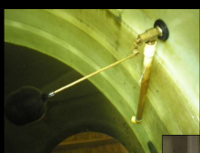
Telescoping Valve. City of Cannon Beach in Clatsop Co. Oregon. 2013.
