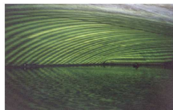
Plate 2.2 - Internal view of a slow sand filter covered by plastic film supported by positive air-pressure at Walton, Thames Water
