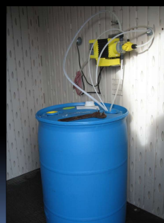
Diaphragm pump with chlorine solution tank
