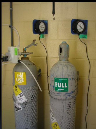
150-lb cylinders Note security chain spare tank & labeling.
