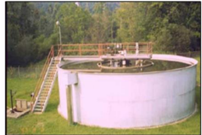
Circular Radial Flow Clarifier
