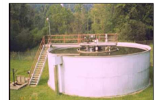
Circular Radial Flow Clarifier
