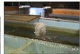
Air binding in a contact adsorption clarifier in California
