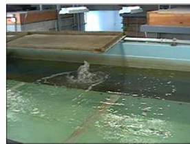
Air binding in a contact adsorption clarifier in California
