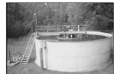
Circular Radial Flow Clarifier
