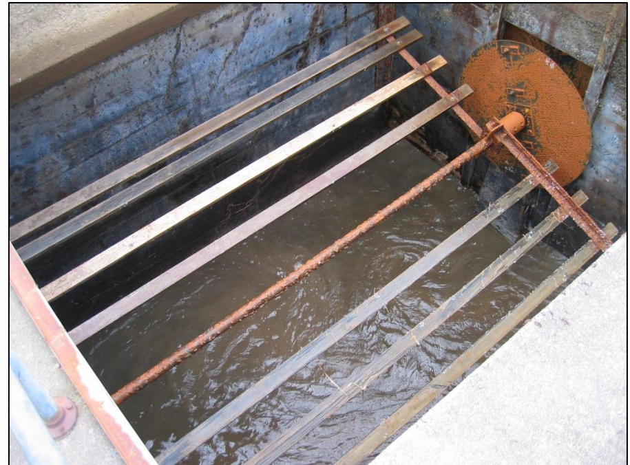
Flocculation paddles - photo from 2007 CPE at Sweethome, OR
