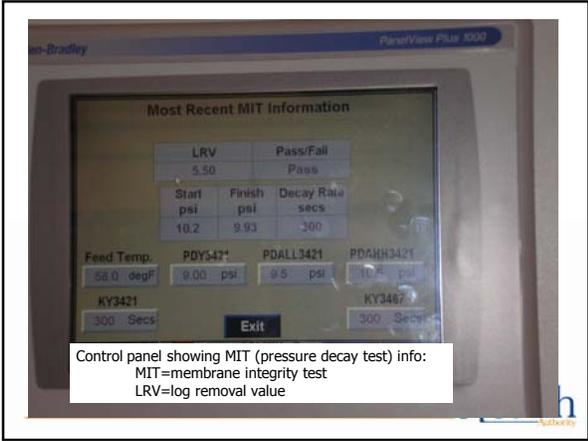
Control panel showing MIT (pressure decay test) info: MIT=membrane integrity test LRV=log removal value
