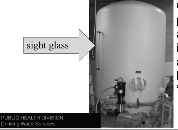
Old style and large pressure tanks have a direct air-water interface that can allow the tank to become "flooded" or "waterlogged".
