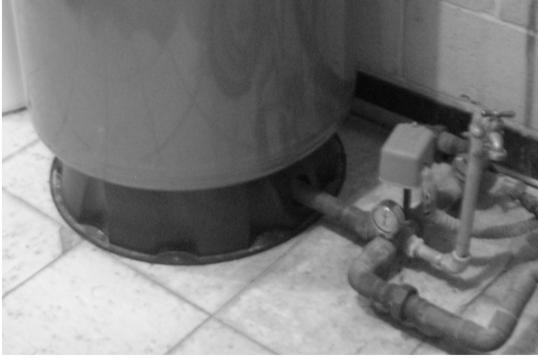
Pressure tanks have "tee" connections so water can always bypass the tank when the well pump runs.
