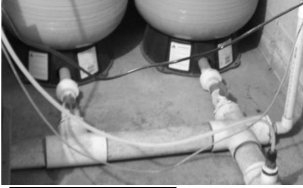
Bladder or diaphragm tanks may need to be disconnected to drain if no tap is near the isolation valve.
