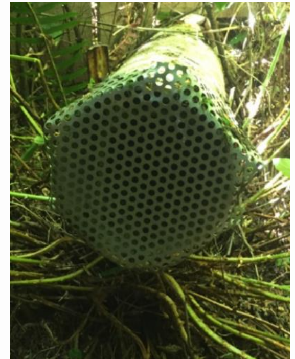
Drain/overflow protected with screen
