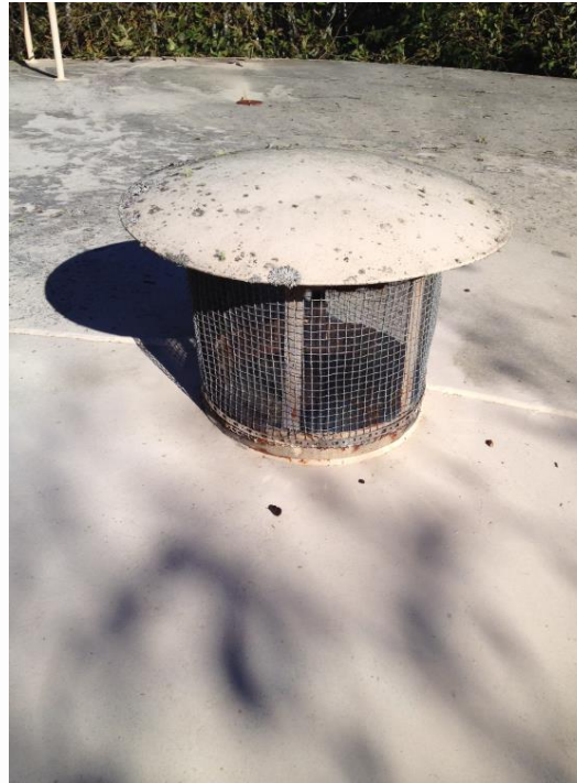
Pic shows the screened vent
