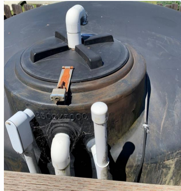
Hatch is secured with lock and watertight
