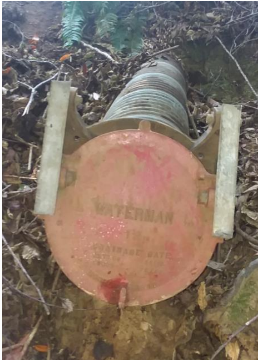
Pic shows the protective flap on drain lines
