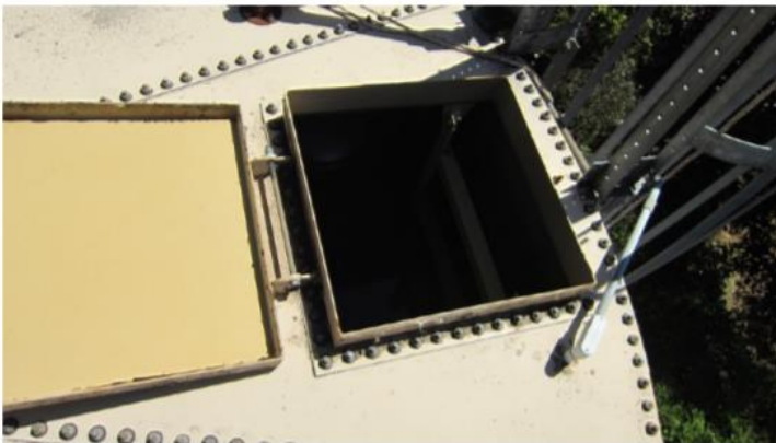
Hatch access to inside of the storage tank - hatch in open position. View to the southwest.
