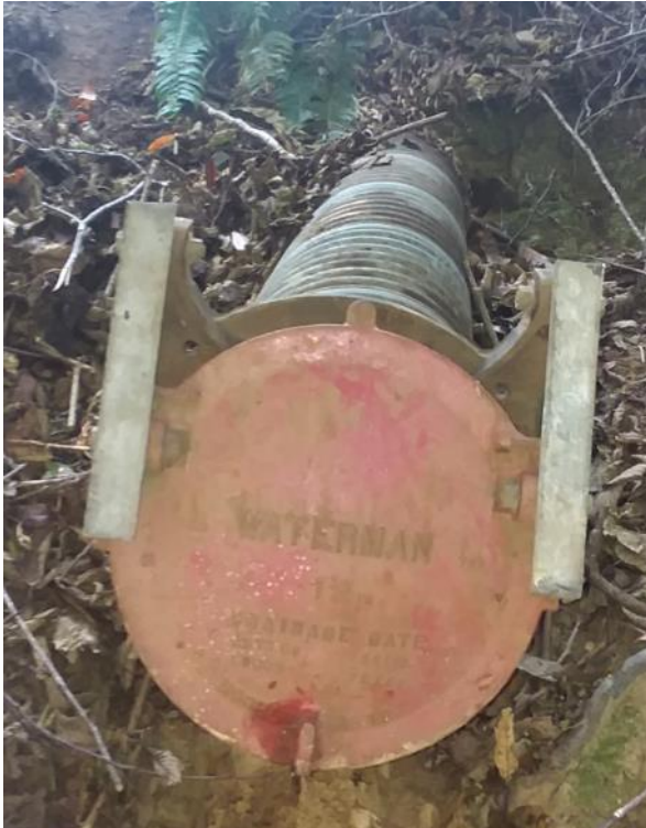
Protective flap on drain line
