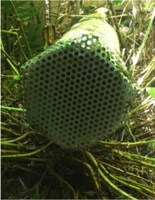
Drain protected with screen
