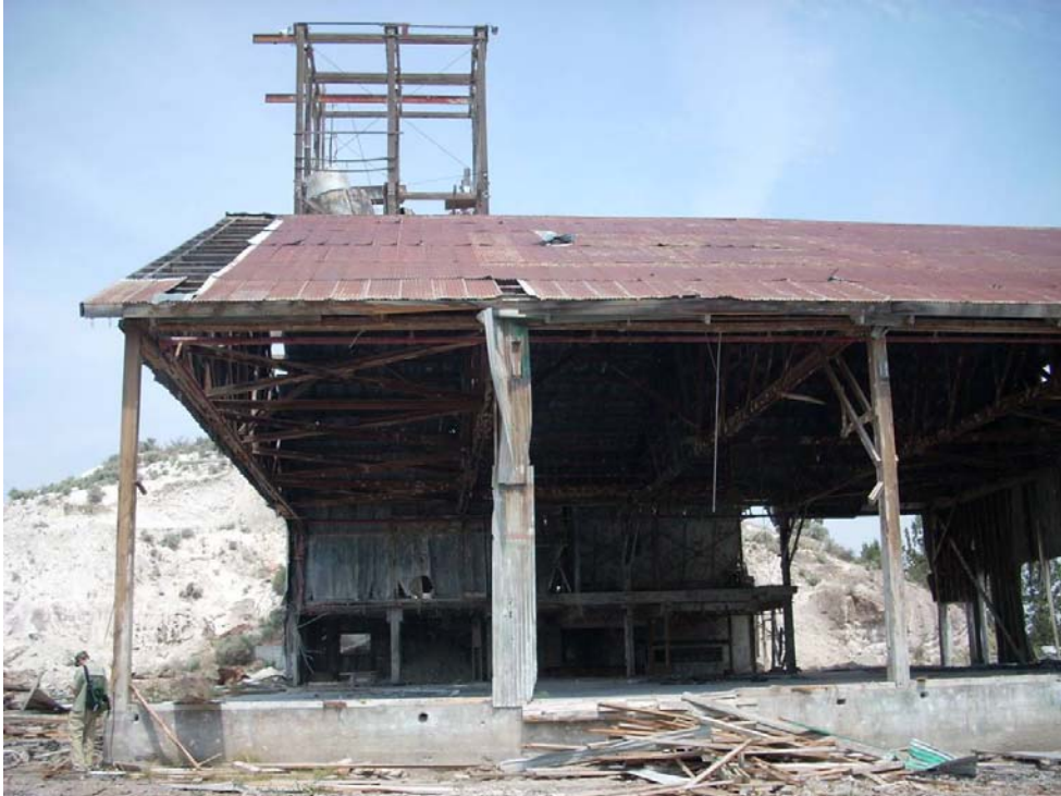
Figure 2. Old mine process building onsite (July 2, 2008; EHAP)
