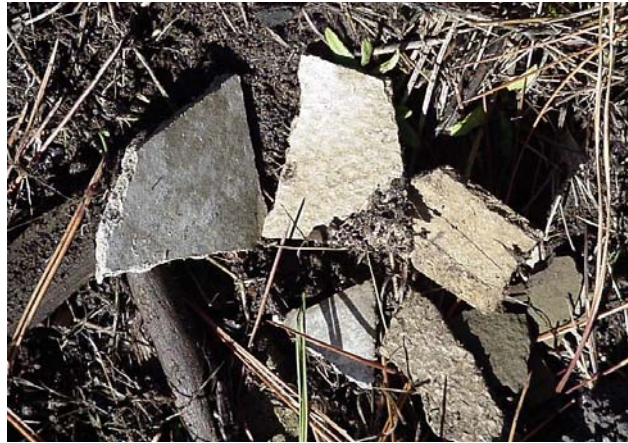
FIGURE 6: CEMENT ASBESTOS BOARD
