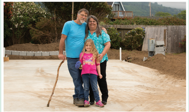
Mike and Collette Bridgeford and granddaughter Sammie Faranda stand on their new home's foundation. They are the fourth Curry County family to get their manufactured home replaced through NeighborWorks Umpqua's reHome Oregon pilot project.
