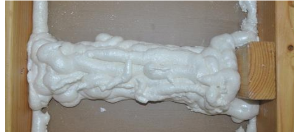
Option 2: Bridge cavities with spray foam
