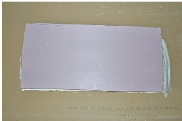
Trim patching material to size and place over sealant
