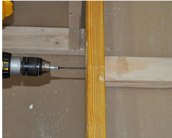
Ensure new bracing is secure by using screws or nails to fasten to the joist
