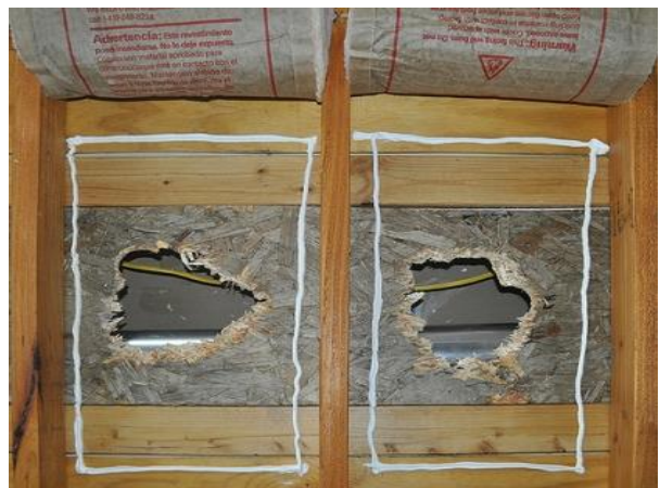
Step 1: Run a bead of sealant around the damaged areas.
