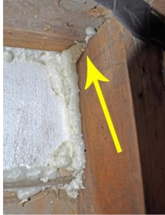
Sealant must be extended along adjacent framing
