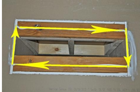
Apply sealant around the opening
