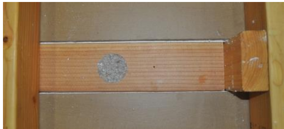
Option 1: Dense pack cavities with cellulose or fiberglass
