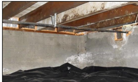
Rim joist insulation & ground cover
