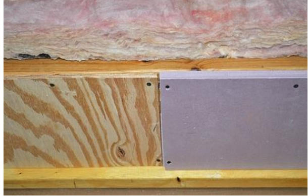
Option 2: Cover the face of the stud bay with rigid material such as XPS or plywood.
