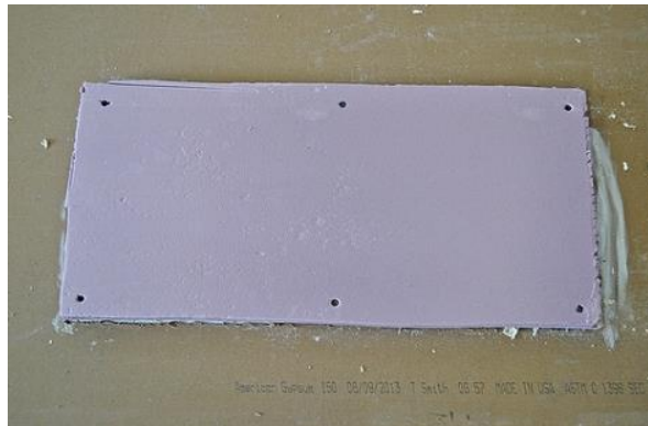
Fasten patching material with screws
