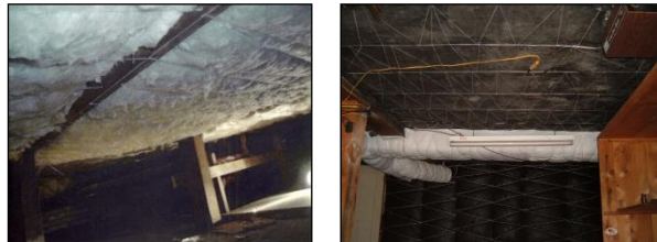
Twining under site built floors
