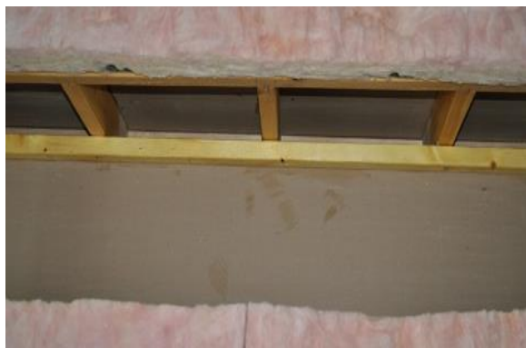
Clear work area of insulation and debris.
