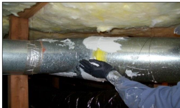
Mastic Being Applied Over Mesh Tape
