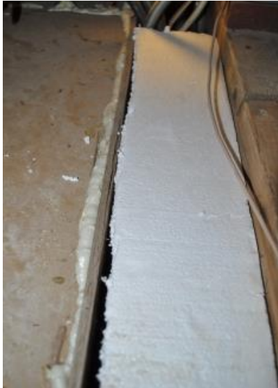
After capping, chases must be sealed
