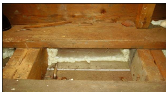
Knee wall blocks needed before insulating
