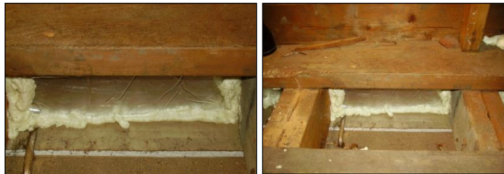
Knee wall block, rigid board insulation secured with foam
