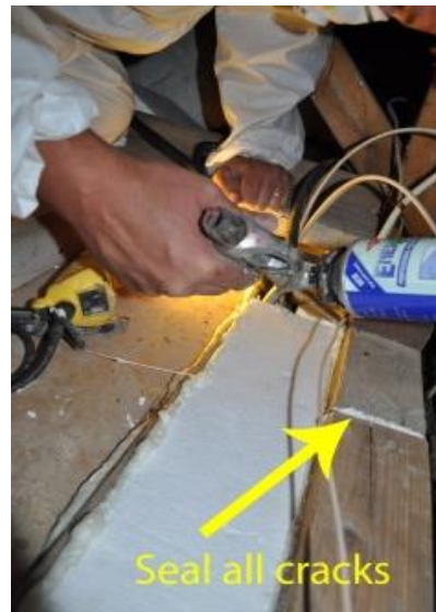
Sealant is used to fill in all cracks and gaps along edges of the cap
