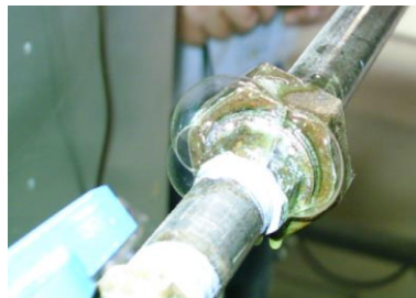
Use soapy water or a gas leak detector to locate leaks.
