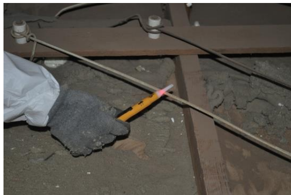
Non-Contact Testing of K&T Wiring
