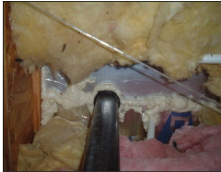
Plumbing penetration sealed
