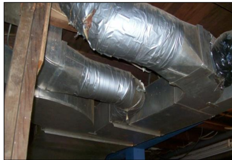
Before Mastic Sealing
