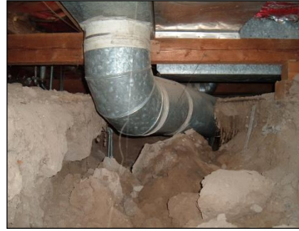
Before Mastic Sealing
