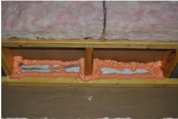
Option 2: Backing used to fill bays and sealed with spray foam.
