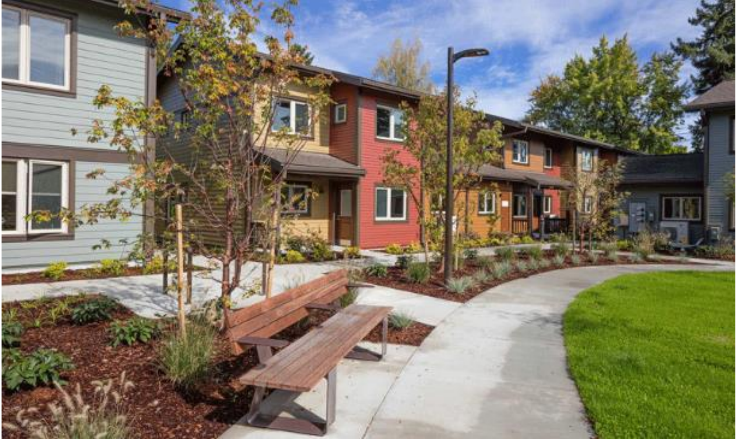
Bridge Meadows Apartments Beaverton, Or
