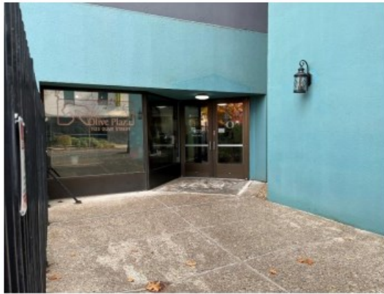
SUBJECT MAIN PEDESTRIAN ENTRANCE
