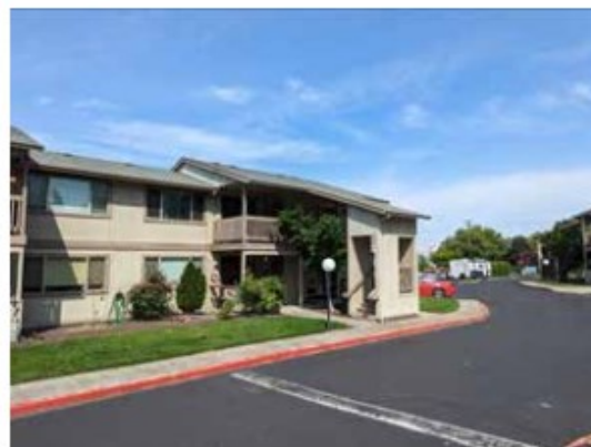
View of subject building exterior and parking areas.
