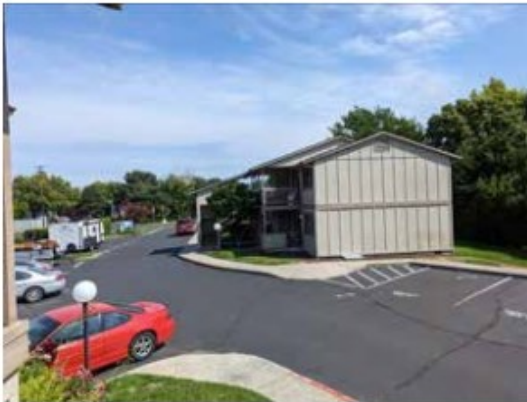
View of subject building exterior and parking areas.
