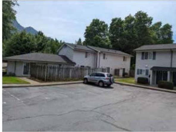
View of subject building exterior.
