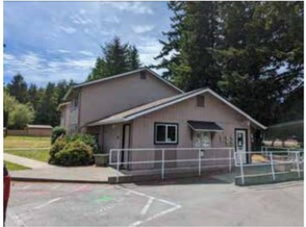
View of subject office/laundry area and apartment building exterior.
