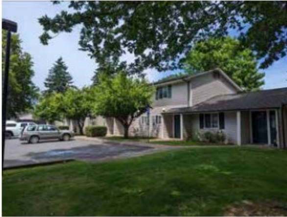
View of subject building exterior.
