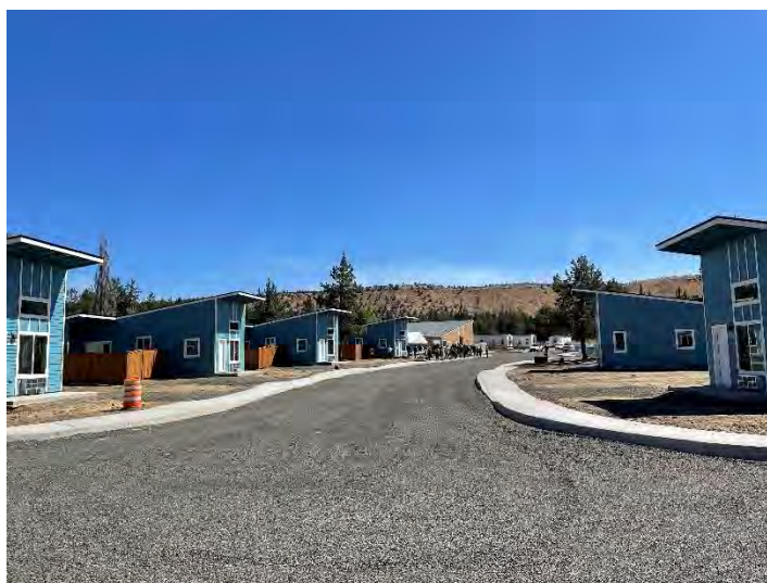
Figure 1 Warm Springs Permanent Supportive Housing Units
