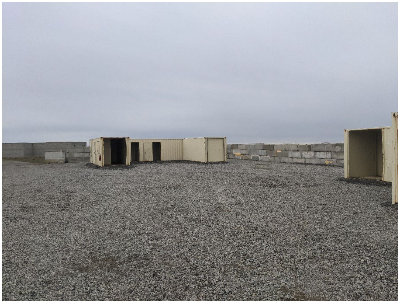
Photo 1: Existing MOUT site at RTC
