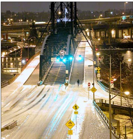
Photo courtesy KATU.com A lone pedestrian negotiates ice covering the Hawthorne Bridge in downtown Portland during ice storms in December, 2006.
