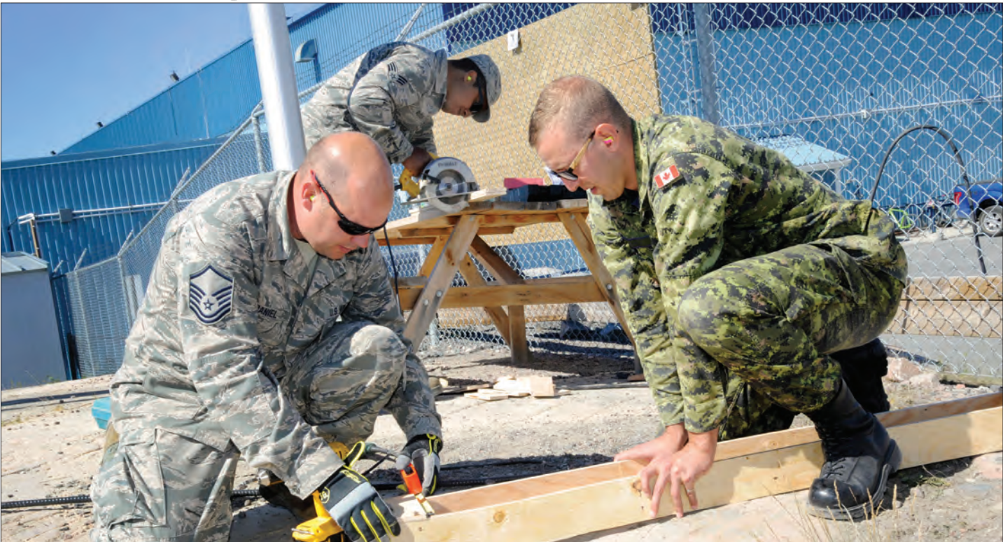
Oregon Air National Guard Master Sgt. Travis McDaniel, a civil engineer assigned to the 142nd Fighter Wing Civil Engineer Squadron and Royal Canadian Air Force Lt. Jordan Vadala, a civil engineer assigned to 4 Wing Cold Lake, construct a concrete form to install a new lighting project at the 440th Squadron, Yellowknife, Northwest Territories, Canada, July 19, 2017.
