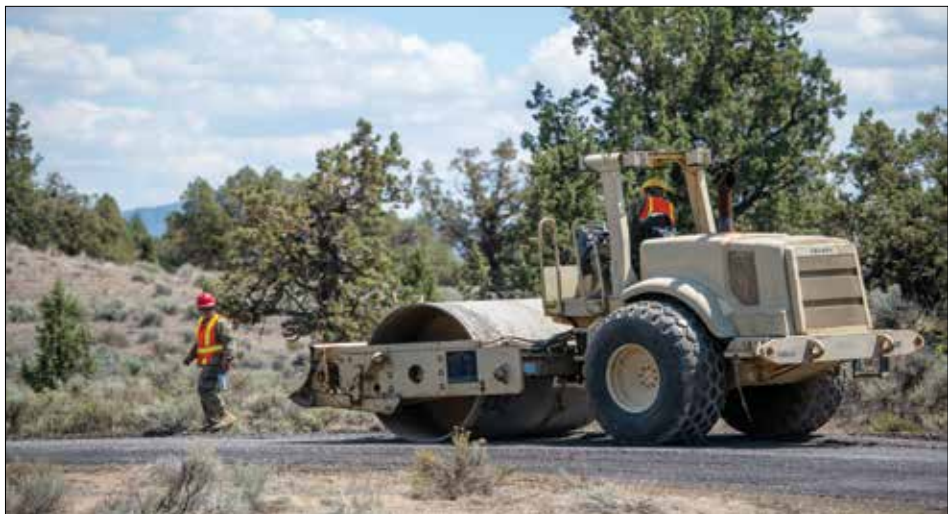
Oregon Army National Guard Soldiers with the 224th Engineer Company, 1249th Engineer Battalion, smooths out a freshly resurfaced road at Biak Training Center near Redmond.
