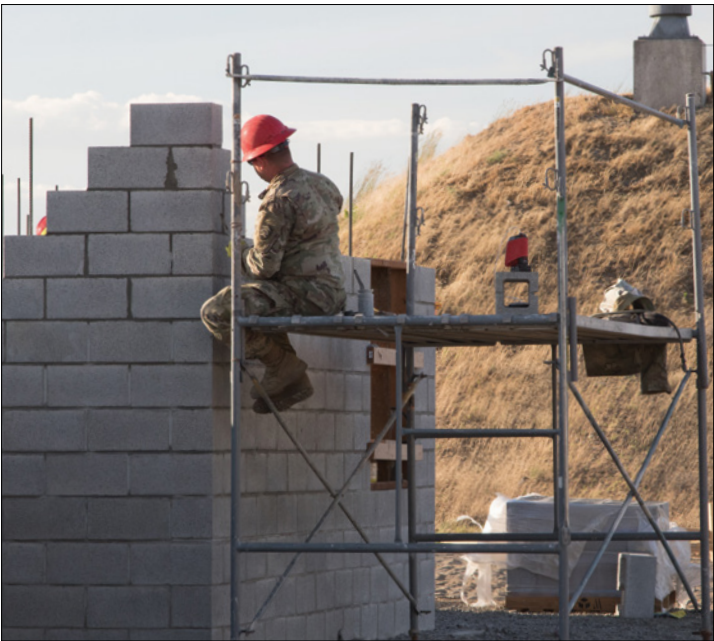
Spc. Gabriel Mischke, 442 Engineers, Oregon Army National Guard, strikes the joint of fresh laid block that will become a permanent three-room shoot house at Camp Umatilla.
