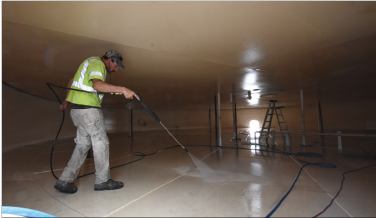
A contractor pressure washes the floor of a massive 600-thousand gallon fuel tank, which stands empty with hatches opened, at the 173rd Fighter Wing in Klamath Falls, Oregon.
