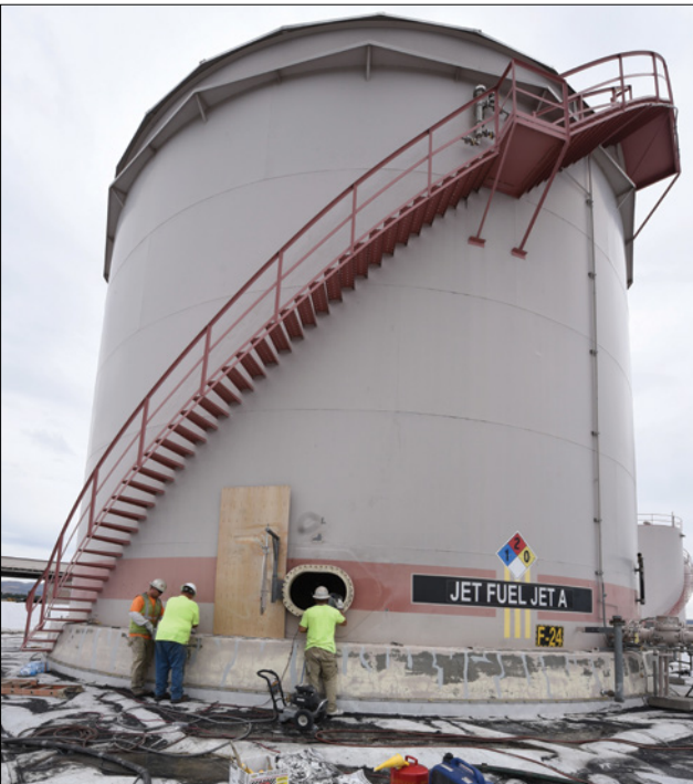
At the 173rd Fighter Wing the main fuel storage tank stands empty for about two weeks while crews perform maintenance to ensure its safe operation for the next decade.
