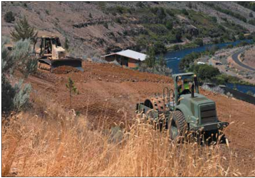
Oregon Army National Guard Soldiers with the 224th Engineer Company, 1249th Engineer Battalion distribute fill with a dozer before using a modified compact roller to build up the ground for the regional high school track improvement project in Maupin, Ore., Aug. 3, 2020.
