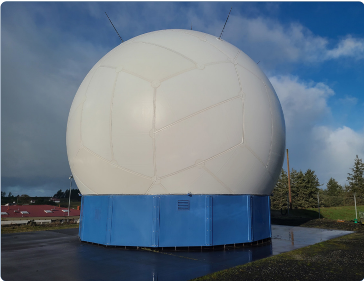
Installation of the 116th Air Control Squadron's new radome structure was completed at Camp Rilea, Warrenton, Ore., on Dec. 13, 2021. Installation of the radome system will protect their TP-75 antenna array against harsh weather conditions on the Oregon Coast and reduce labor by 300 man-hours annually.
