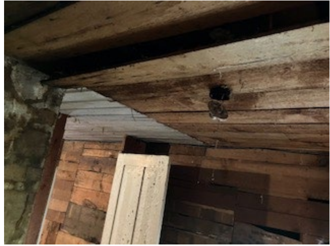
Ceiling light fixture to be updated. (chimney to left)
