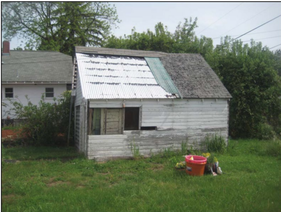
Photo 2 of 2: Amendment_OR_BentonCounty_HannahandElizaGormanHouse_0002 Overview of Garage, camera facing north.
