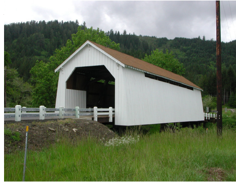
Hayden Bridge, Benton County
