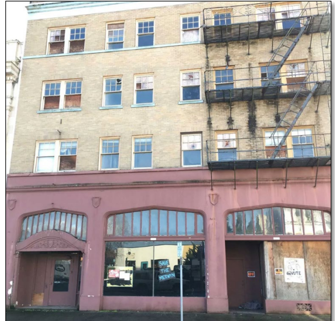
MERWYN BUILDING BEFORE REHABILITATION IN DOWNTOWN ASTORIA.
