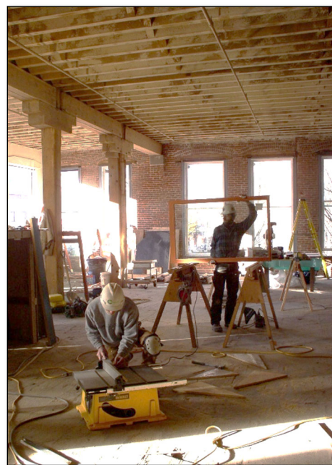
WINDOW REHABILITATION WAS A PART OF THE APPROVED SCOPE OF WORK FOR THE SKIDMORE BLOCK.
