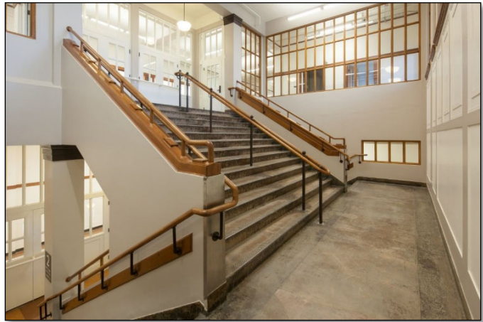
IN COORDINATION WITH SHPO, COMPATIBLE NEW HANDRAILS AND GUARDRAIL EXTENSIONS WERE DESIGNED TO MEET THE SECRETARY'S STANDARDS IN THIS HISTORIC HIGH SCHOOL BUILDING.
