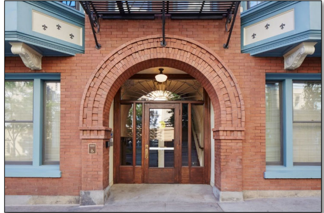
THE BRONAUGH APARTMENTS INCLUDED SEISMIC UPGRADE MEASURES THAT SEAMLESSLY TIED THE EXTERIOR BRICK TO THE OVERALL STRUCTURE, USING APPROVED MEASURES THAT DID NOT VISUALLY COMPROMISE THE EXTERIOR CHARACTER.
