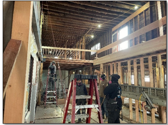
WORKERS BUILD A NEW ELEVATOR CORE WITHIN THE WAUCOMA HOTEL.
