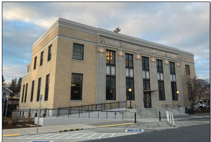
AN ADA RAMP AT THIS HISTORIC POST OFFICE BUILDING WAS CONSTRUCTED TO ONE SIDE OF THE ENTRANCE.
