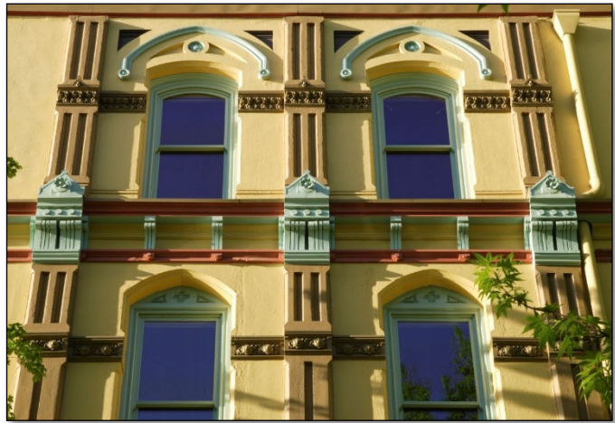
DUE TO HEAVY DETERIORATION, NEW CUSTOM WOOD WINDOW SASHES WITH INSULATED GLAZING UNITS WERE APPROVED FOR REINSTALLATION IN THE REFURBISHED WOOD FRAMES AT THE BICKEL BLOCK.
