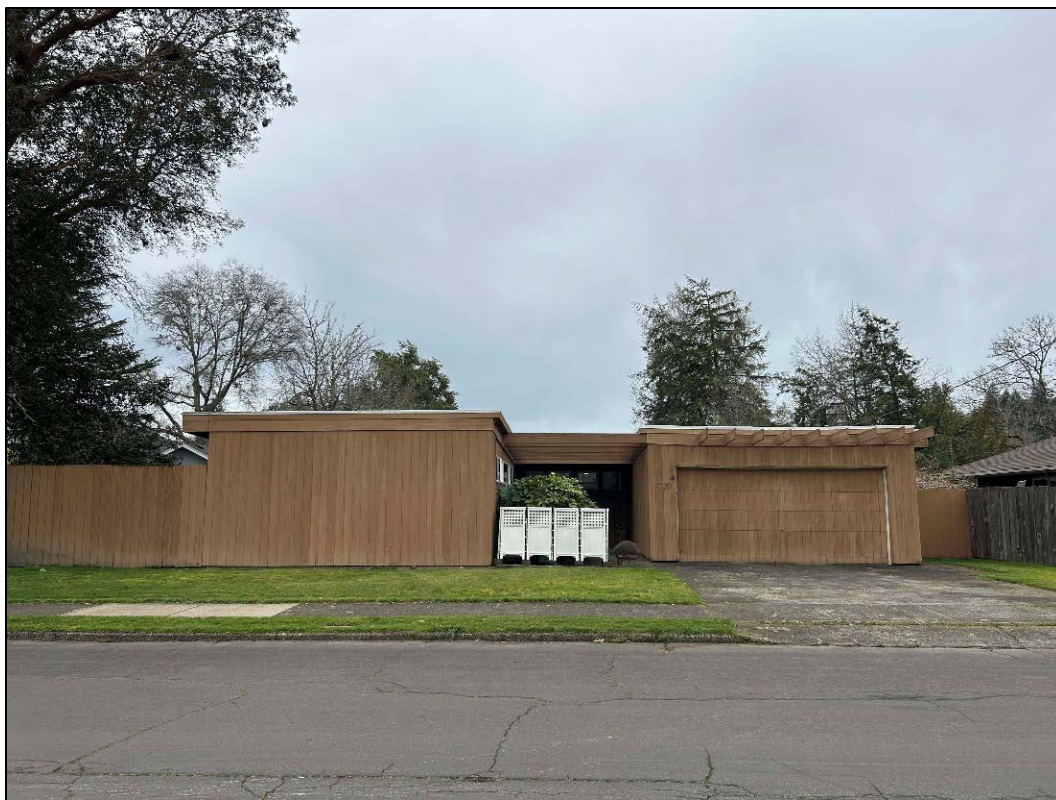
Photograph 1 of 16: OR_BentonCounty_YangEdithHouse_0001 The Edith Yang House façade, view facing west.
