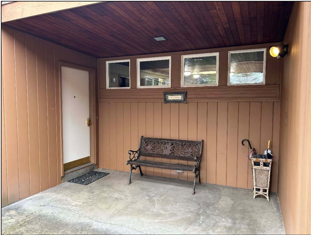
Photograph 3 of 16: OR_BentonCounty_YangEdithHouse_0003 The Edith Yang House entry courtyard, view facing southwest.
