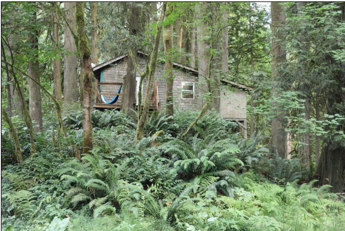
Photo 2 of 20: OR_ClackamasCounty_CampNamanu_0002 North façade of Trillium Cottage, including the entry, looking south
