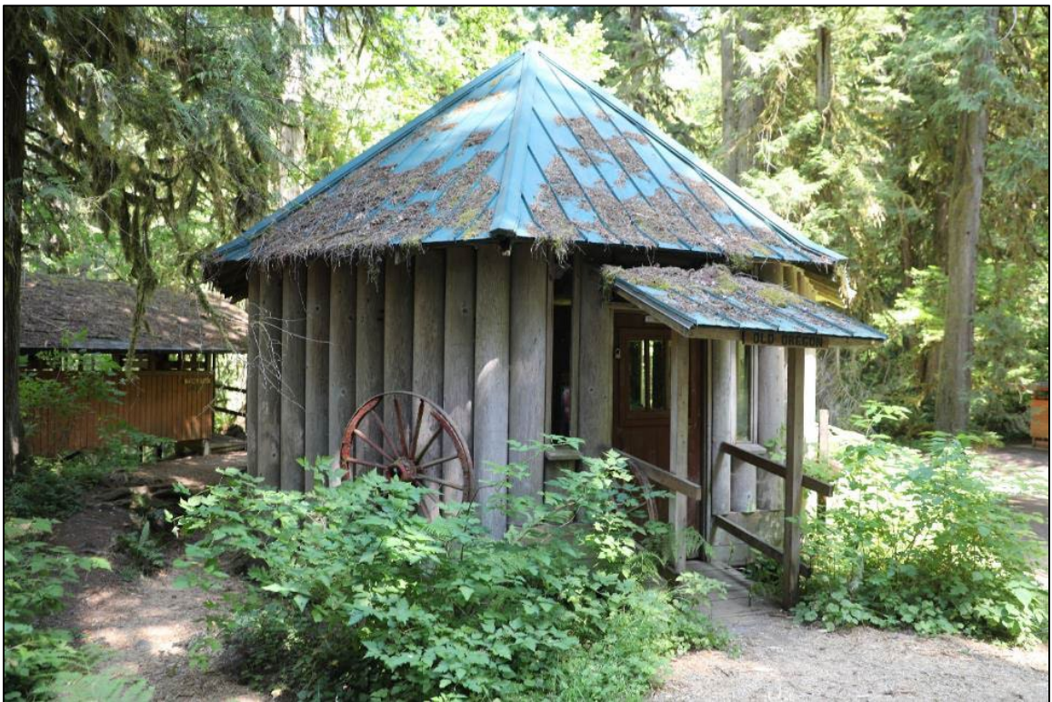
Photo 14 of 20: OR_ClackamasCounty_CampNamanu_0014 Old Oregon Lodge at the Riverbend Cabins Cluster, looking north
