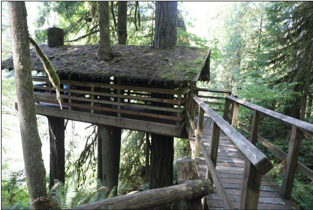
Photo 15 of 20: OR_ClackamasCounty_CampNamanu_0015 The footbridge approach to Coho sleeping cabin in the Balagan Cabin Cluster, looking northwest
