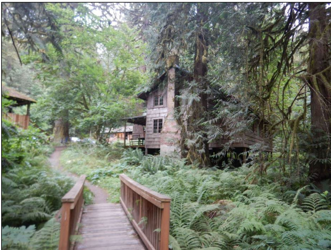
Photo 20 of 20: OR_ClackamasCounty_CampNamanu_0020 Another footbridge located in Administrative Cluster; the north façade of Guardians Lodge is visible in the background, looking south
