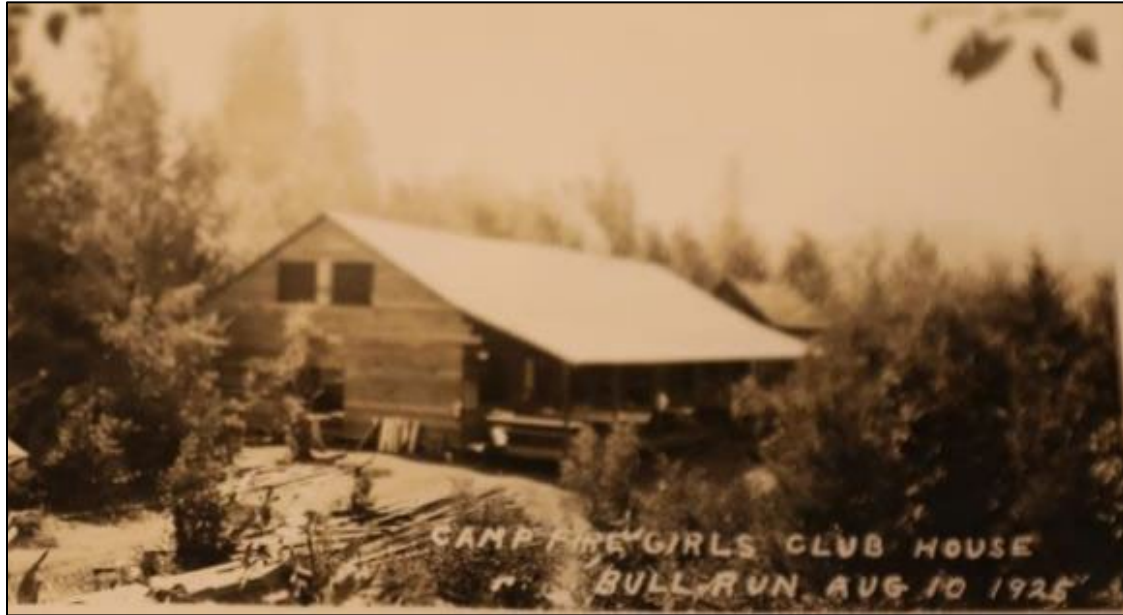
Figure 9: Construction on the original Raker Lodge (non-extant) in 1925, designed by A.E. Doyle. Courtesy Camp Namanu archives.
