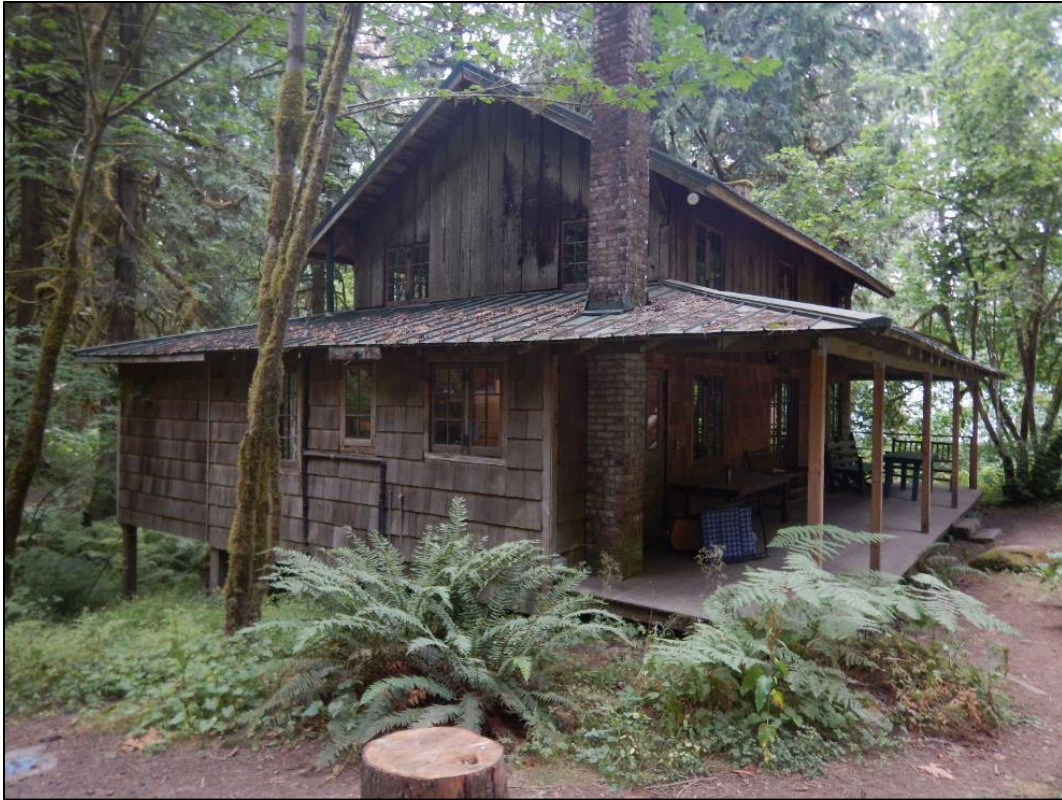
Photo 5 of 20: OR_ClackamasCounty_CampNamanu_0005 Secondary façade at Guardians Lodge, looking north
