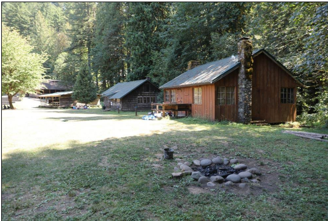
Photo 6 of 20: OR_ClackamasCounty_CampNamanu_0006 A view of the buildings at the south end of the Meadow Cluster: Cobb Cottage, the Weavery, and the Craft Barn, looking southeast
