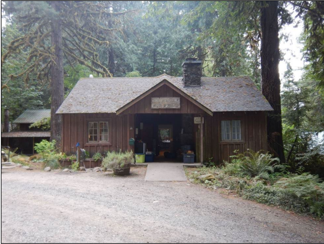
Photo 3 of 20: OR_ClackamasCounty_CampNamanu_0003 North Primary façade of Camp Office (formerly known as the House of Health or House of Help) with entry porch, looking west
