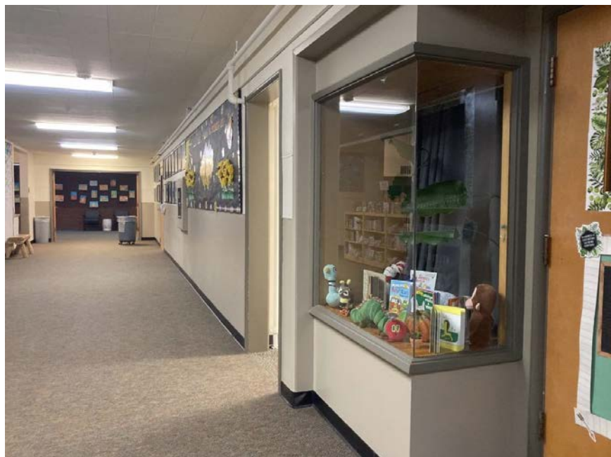
Photograph 26 of 69: OR_ClackamasCounty_BoltonSchool_0026 Interior, corridor of the 1950 classroom wing, detail of original built-in display window in active use. Camera facing southeast.
