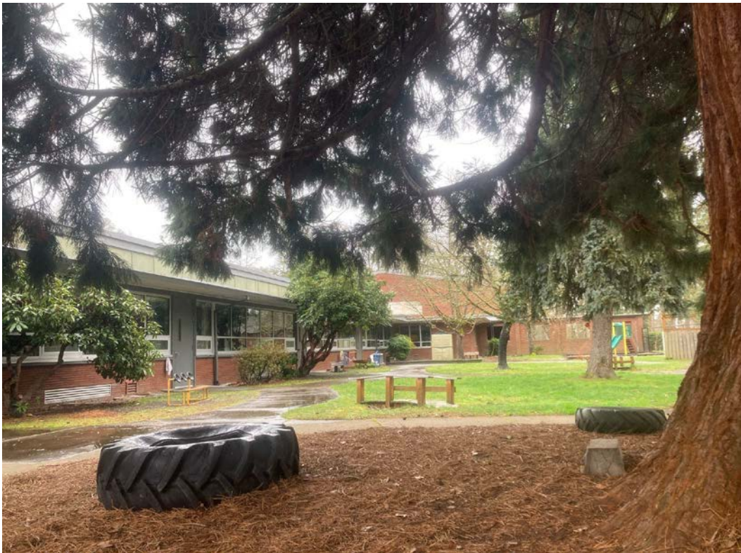
Photograph 4 of 69: OR_ClackamasCounty_BoltonSchool_0004 Looking west at main entrance and classroom wing from kindergarten playground from beneath mature cedar tree.
