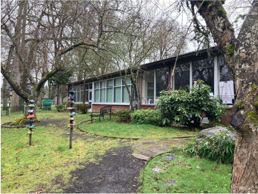
Photograph 5 of 69: OR_ClackamasCounty_BoltonSchool_0005 Looking southeast at rear classroom wing from Perrin Street easement, Hammerle Park grounds continuous.
