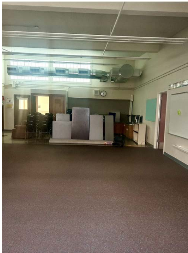
Photograph 16 of 69: OR_ClackamasCounty_BoltonSchool_0016 Interior, classroom in the 1965 addition, showing glass-block monitor glazing in service above surface-mounted mechanical ductwork installed 2021. Camera facing northeast.
