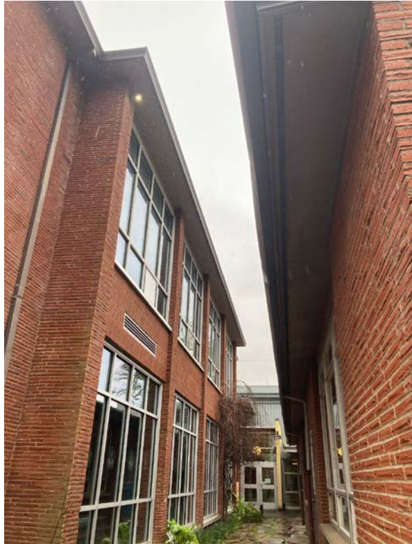
Photograph 7 of 69: OR_ClackamasCounty_BoltonSchool_0007 Looking northwest through the exterior passage between the cafeteria volume and the 1965 classroom addition.
