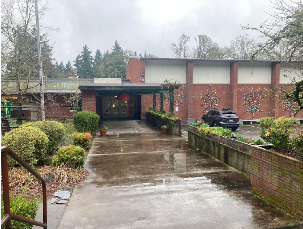
Photograph 1 of 69: OR_ClackamasCounty_BoltonSchool_0001 Looking northeast at southwest (primary) façade, primary entrance and gymnasium. Compare with Figure 47 for front entrance after secure remodel.
