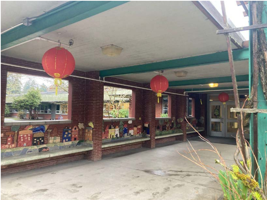
Photograph 3 of 69: OR_ClackamasCounty_BoltonSchool_0003 Looking north from under the entrance canopy, bricked openings with built-in benches decorated in ceramic tile mural and main entry doors.
