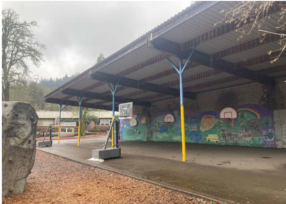
Photograph 15 of 69: OR_ClackamasCounty_BoltonSchool_0015 Looking south at 1957 covered play shed (contributing structure).
