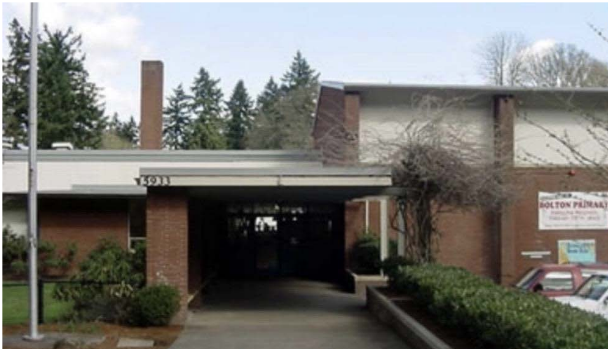
Figure 46. Front entrance per district 2008 bond website before secure front entrance remodel www.bond.wlwy.k12.or.us , wayback machine, archived 2012, compare with Photograph 1.
