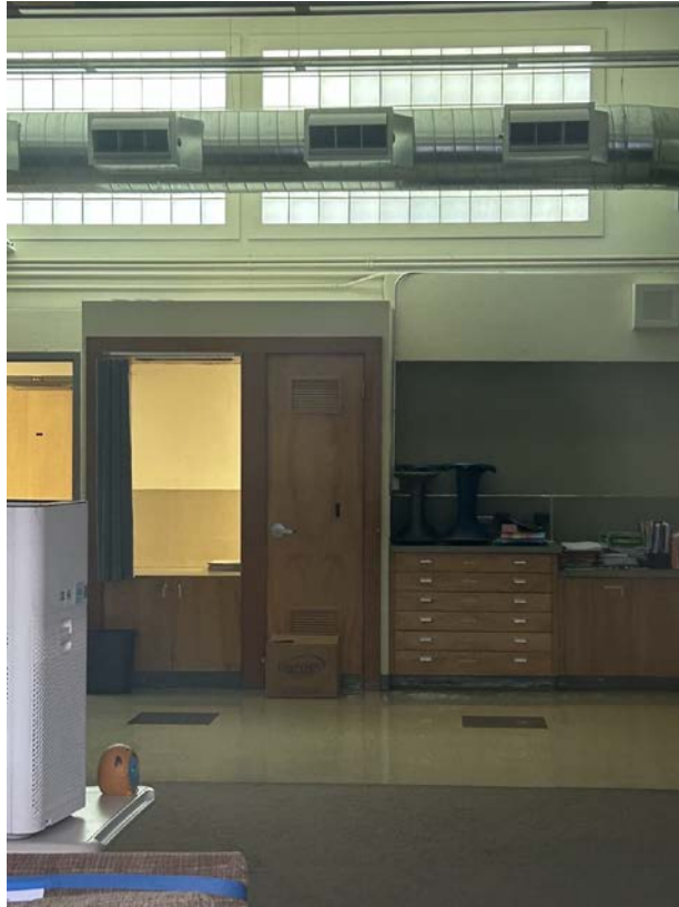
Photograph 25 of 69: OR_ClackamasCounty_BoltonSchool_0025 Interior, classroom in the 1965 addition, showing original built-in cabinetry, flat-file drawers, and counter; glass-block monitor glazing in service above with surface-mounted mechanical ductwork installed 2021. Camera facing northeast.
