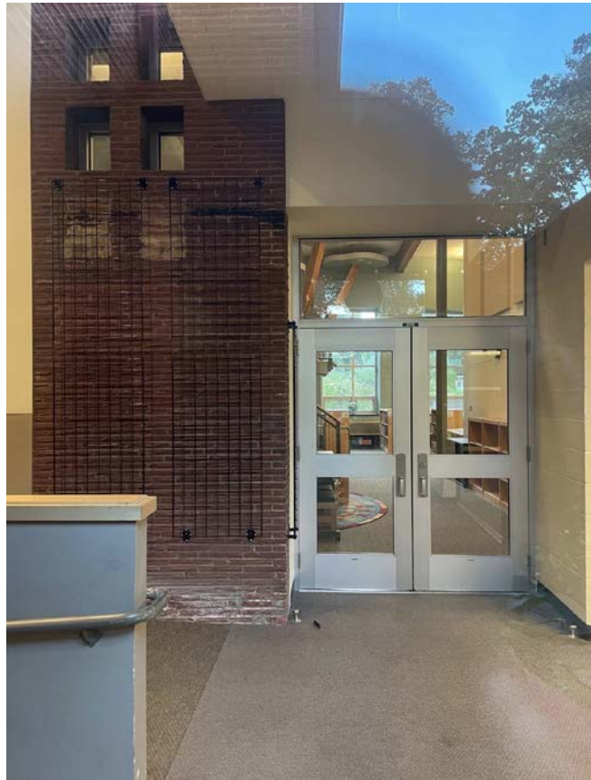
Photograph 33 of 69: OR_ClackamasCounty_BoltonSchool_0033 Interior, circulation space at the 2012 library addition, showing the original exterior perforated brick pier and wall surfaces preserved in place within the addition. Camera facing northwest.
