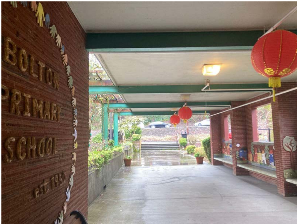
Photograph 2 of 69: OR_ClackamasCounty_BoltonSchool_0002 Looking southwest from entrance canopy toward Willamette Drive (Highway 43), "BOLTON PRIMARY SCHOOL EST. 1950" lettering visible.
