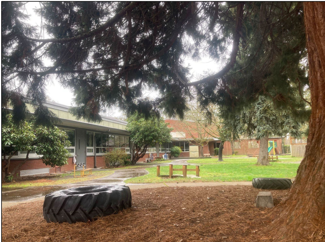
Photograph 4 of 15: OR_ClackamasCounty_BoltonSchool_0004 Looking west at main entrance and classroom wing from kindergarten playground from beneath mature cedar tree.
