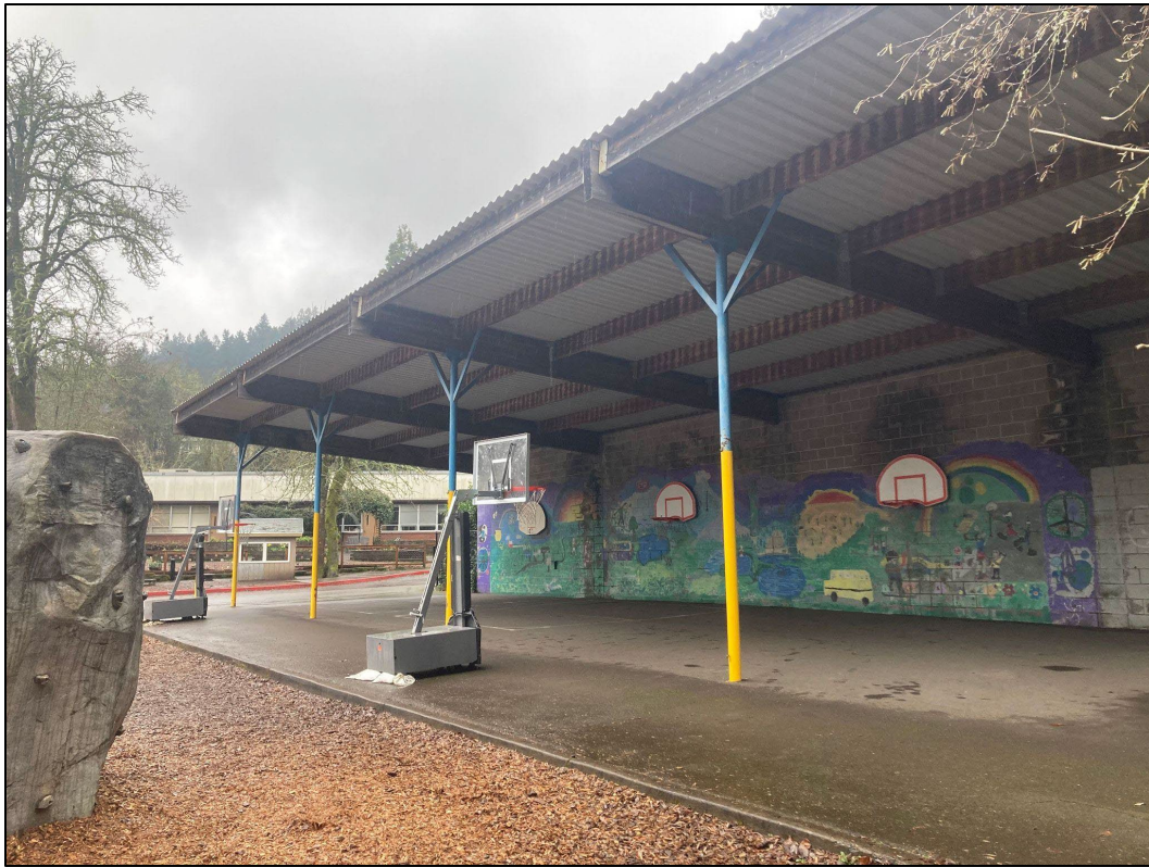
Photograph 15 of 15: OR_ClackamasCounty_BoltonSchool_0015 Looking south at 1957 covered play shed (contributing structure).
