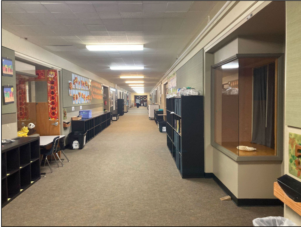
Photograph 11 of 15: OR_ClackamasCounty_BoltonSchool_0011 Interior, looking southeast along main level corridor with built-in display windows.
