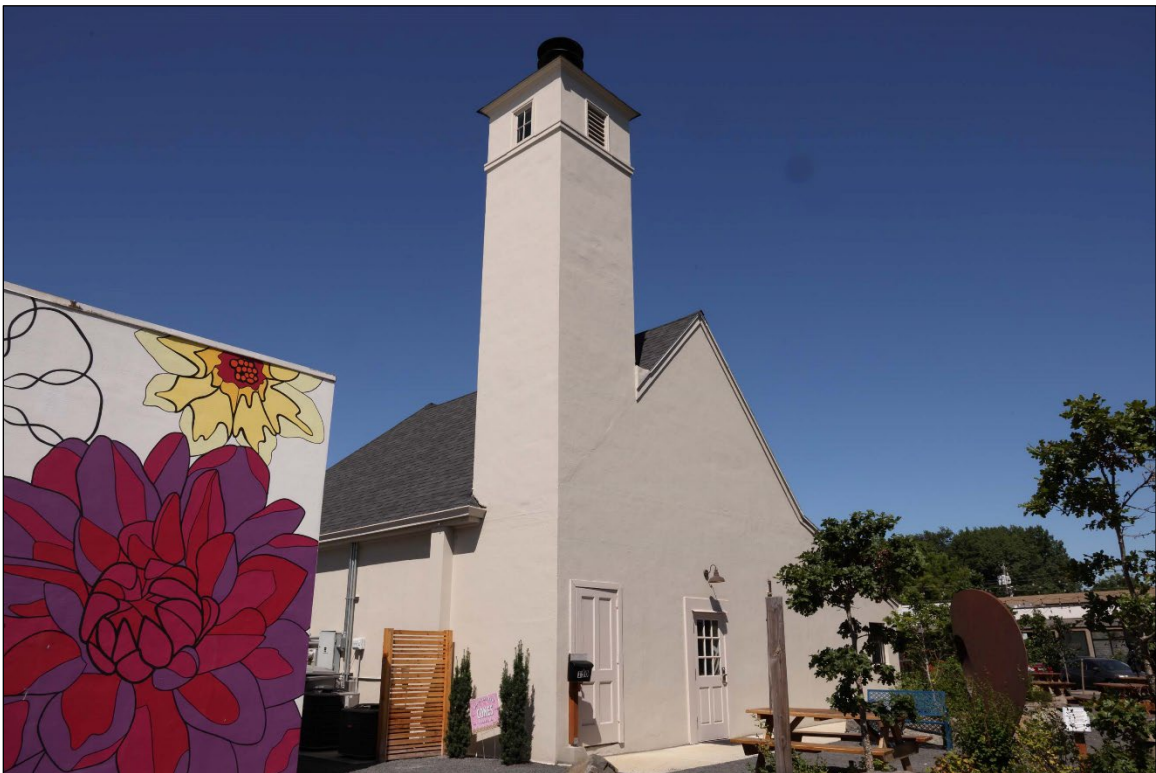
Photograph 8 of 14: OR_ClackamasCounty_CanbyCityHall_0008 Oblique view of firehouse showing south and east façades, camera facing north-northwest.
