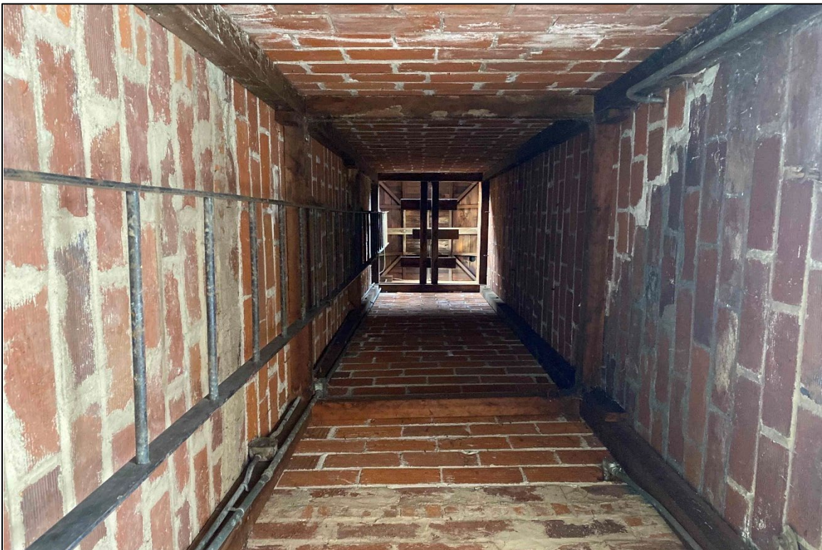
Photograph 14 of 14: OR_ClackamasCounty_CanbyCityHall_0014 Interior of hose tower, facing up.
