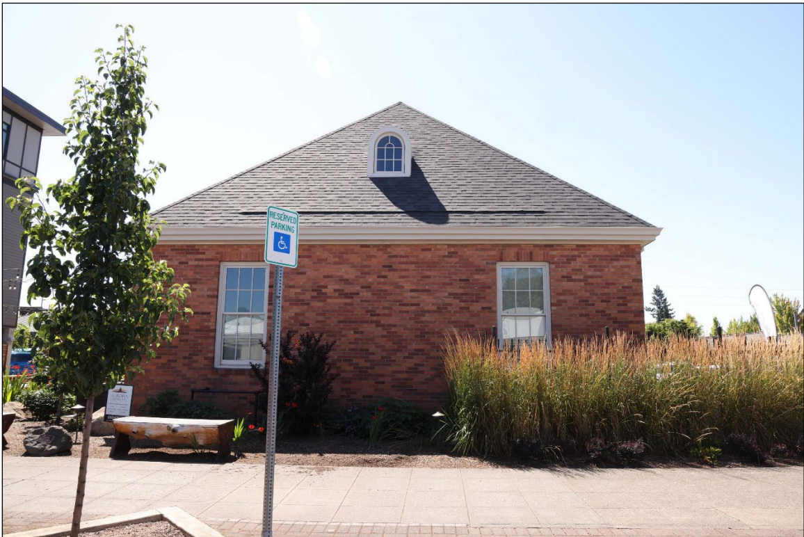
Photograph 4 of 14: OR_ClackamasCounty_CanbyCityHall_0004 North façade of main volume, camera facing south-southeast.
