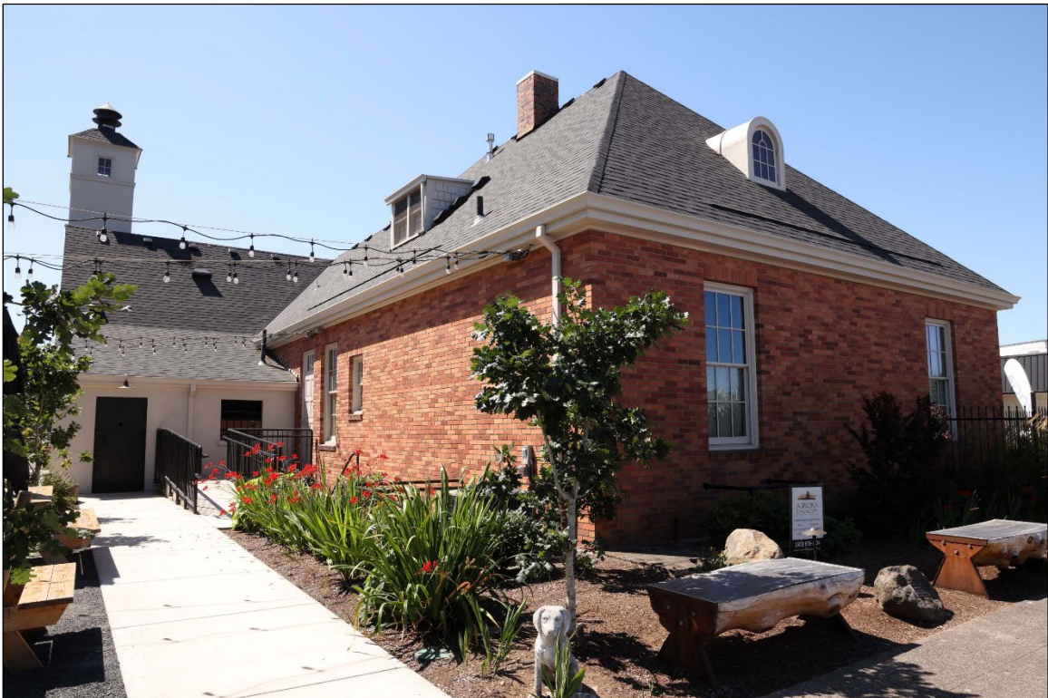
Photograph 6 of 14: OR_ClackamasCounty_CanbyCityHall_0006 Oblique view of east and north façades, camera facing south.
