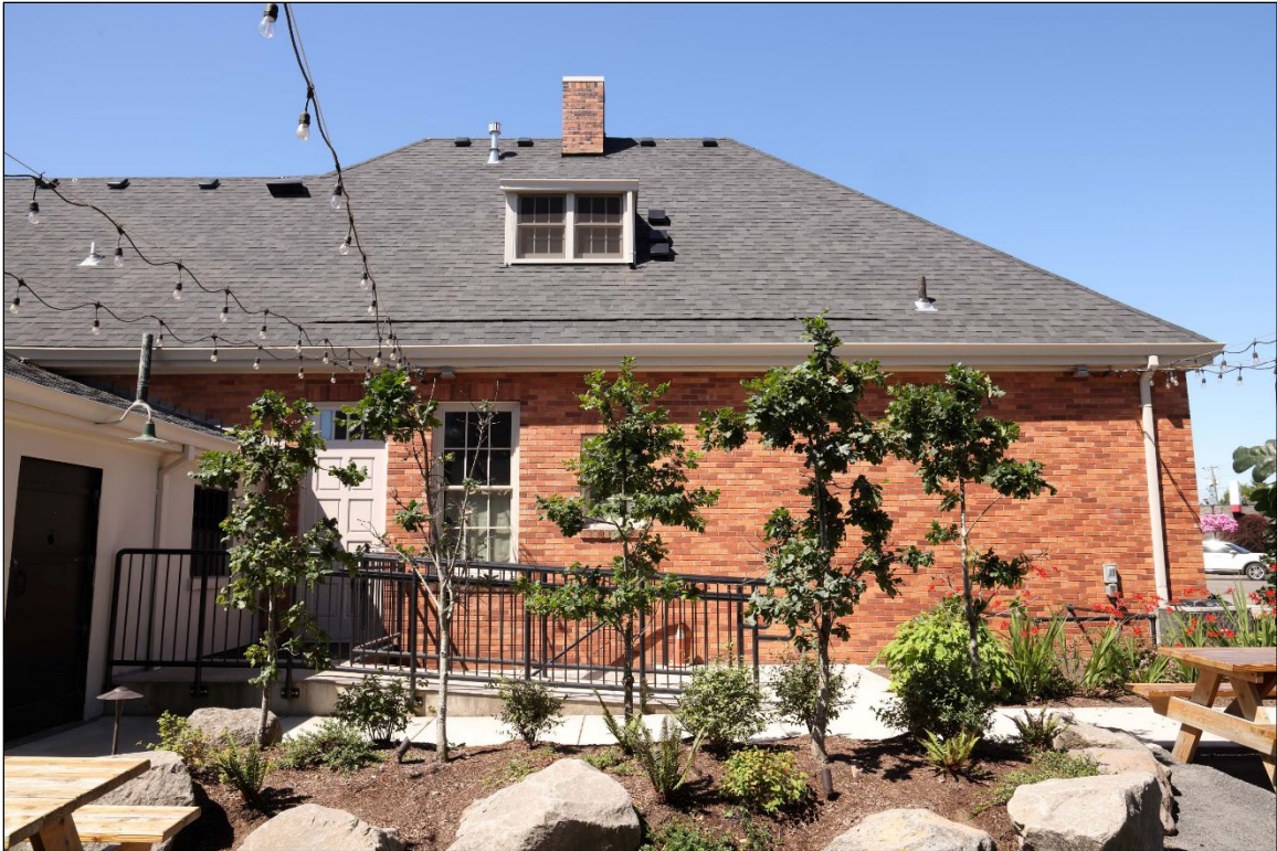
Photograph 5 of 14: OR_ClackamasCounty_CanbyCityHall_0005 East façade of main volume, camera facing west-southwest.
